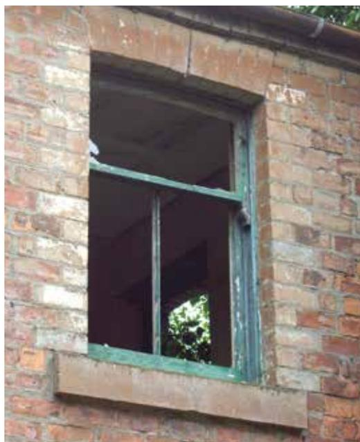
*Window frames which appear to be in poor condition are not necessarily beyond repair.*
