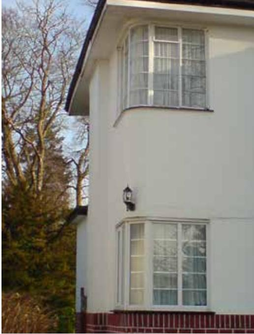
*On close inspection the chunky uPVC frame on the ground floor is incapable of replicating the elegance of the original Crittal window frames and curved glass above on this 1930s Art Deco house.*
