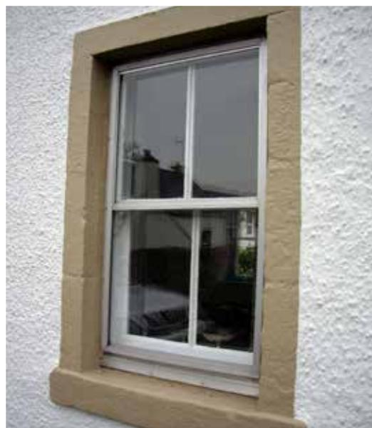
*This window features an external secondary glazing system designed so that the original window can still be seen clearly.*
