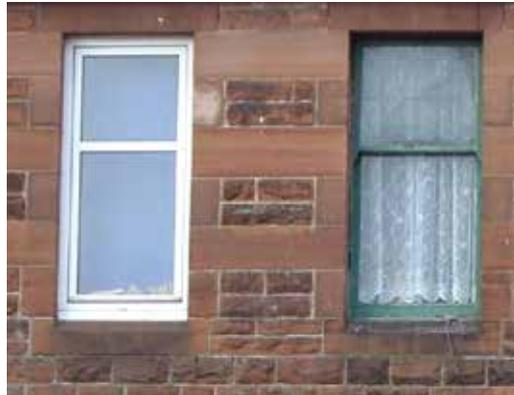
*The replacement uPVC windows differ from the originals in material, design, colour, profile and opening method—this cannot be considered 'like for like'.*
